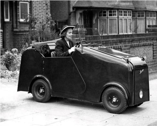
Even the diminutive Peel P-50, recognized as the world's smallest car, is over 1 ft. wider than the Larmar. Besides its narrow width the Larmar was well-engineered, with 4-wheel independent suspension, easy hand starting, and a very short 15 ft. turning circle.
